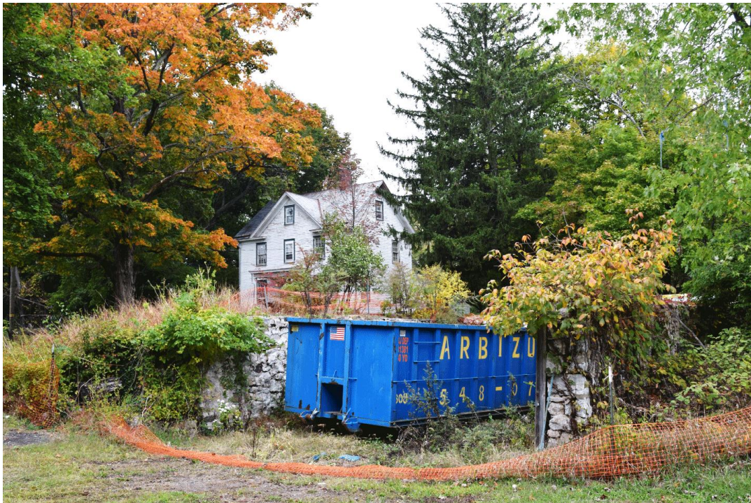
Image 17: Cattle Barn Foundation
