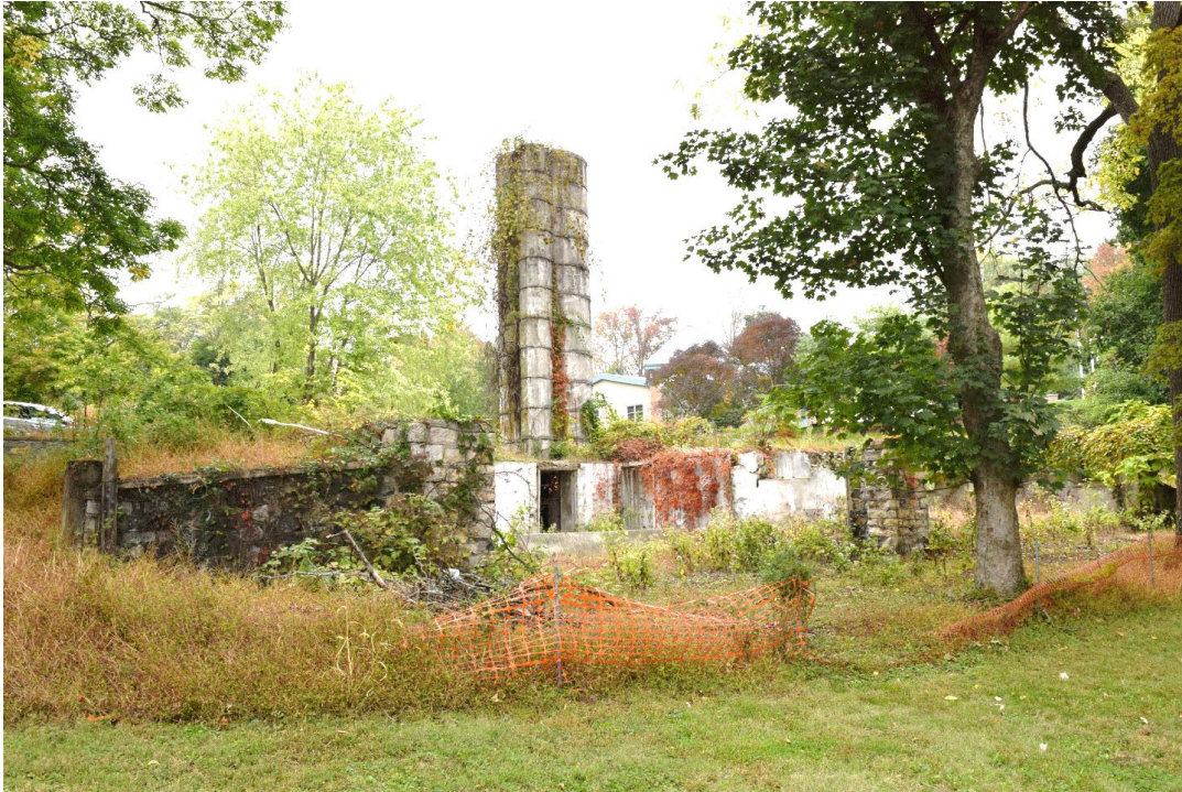
Image 16: Dairy Barn Foundation and Silo
