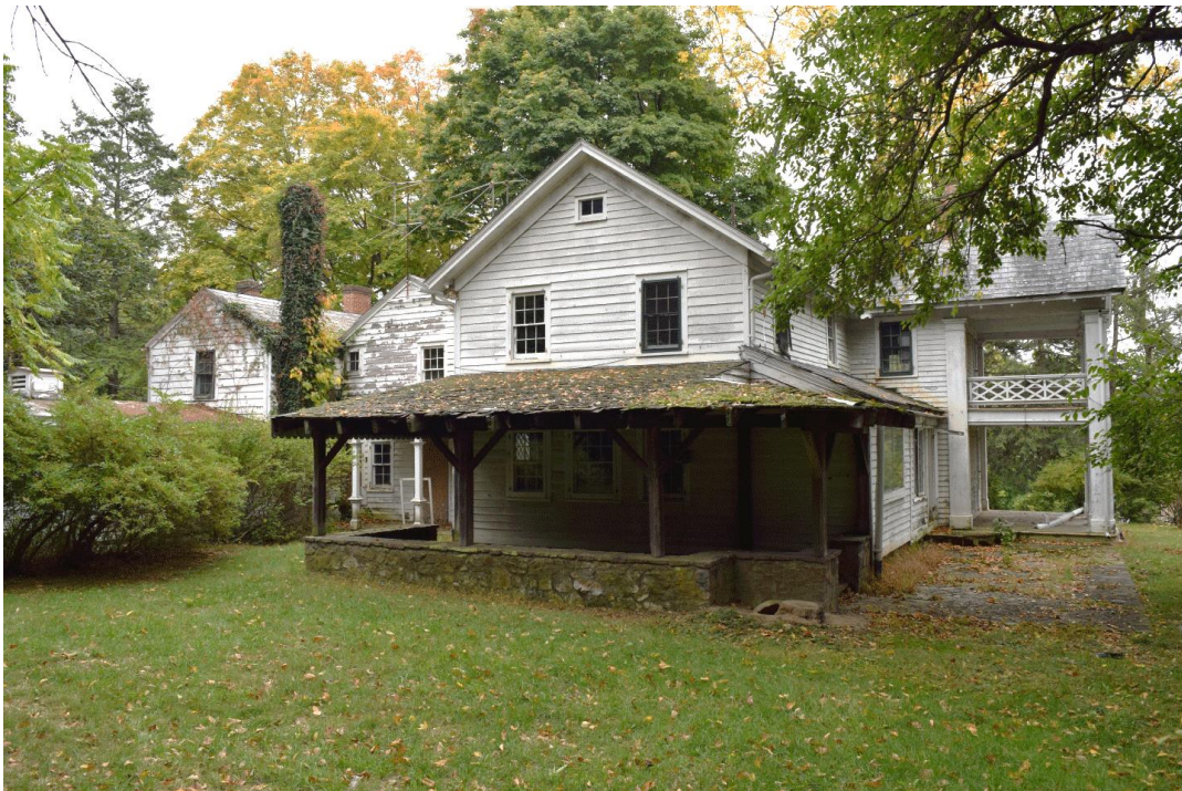
Image 4: Rear of the Main House
