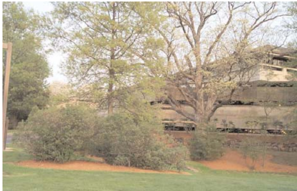
The rear facade of this building has as much detail as front facade. Mechanical equipment is well screened.
